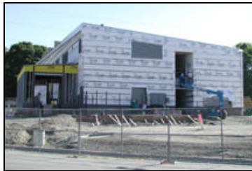
Southwest Precinct, under construction. The facility is now finished.
